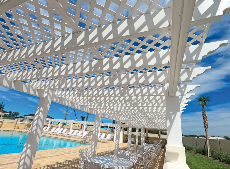
DuraShell® diagonal lattice application utilizing H-Channel and U-Channel in a commercial pergola project.
